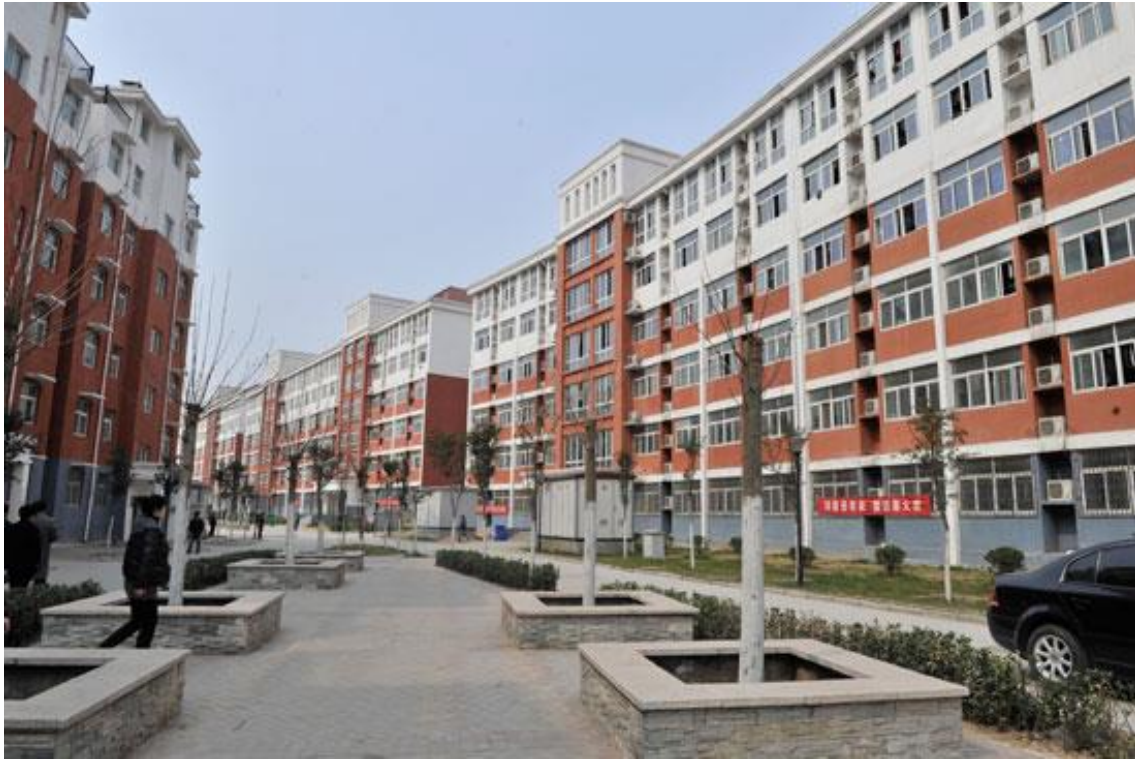
Figure 6-8 Xinzheng Foxconn Airport Staff Apartment Dormitory Area
